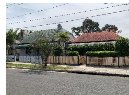
Figure 5.4 44–46 Kings Road (listed).
