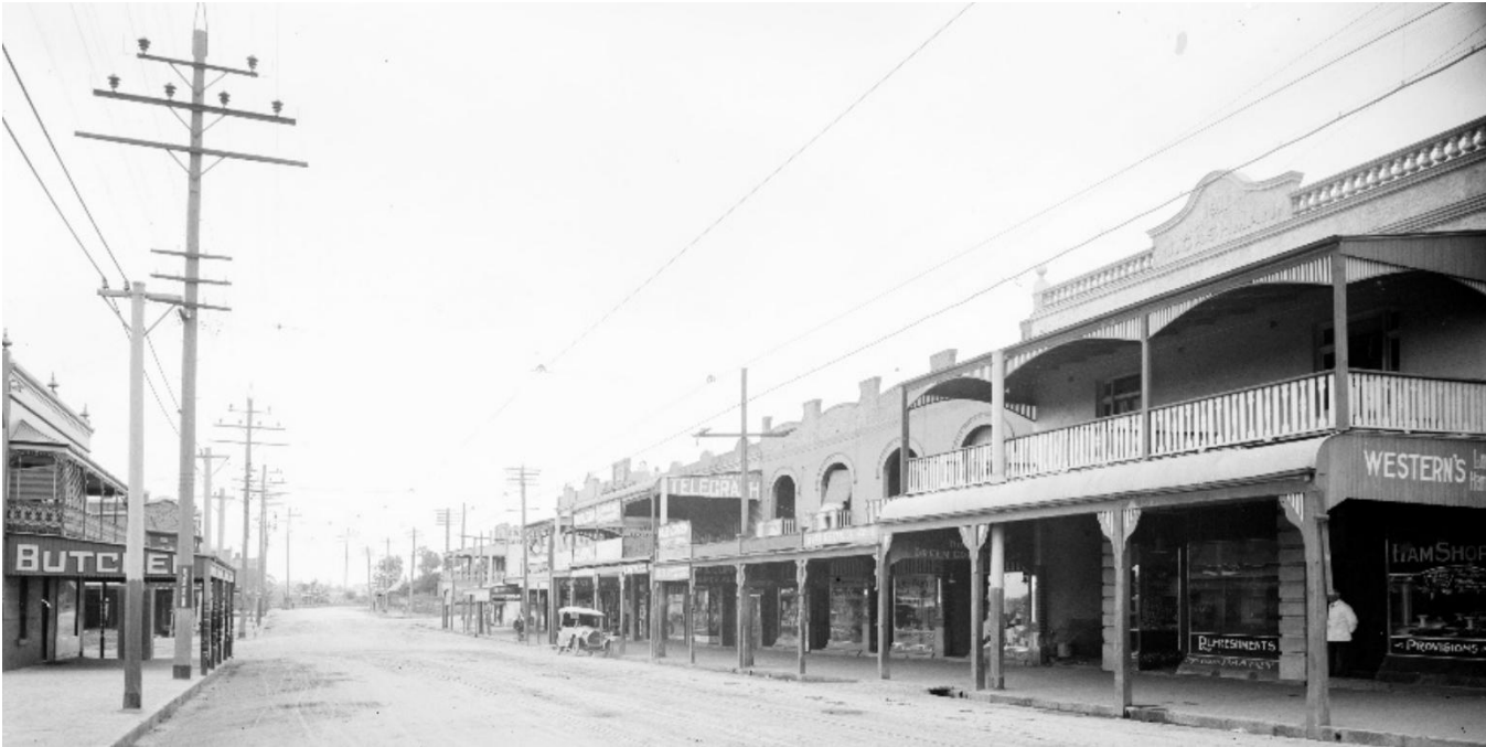
Figure 4.8 Great North Road, looking south from the Garfield Street intersection in the twentieth century, prior to the construction of Five Dock Hotel on left. (Source: Ernest Foster, SLNSW, FL400575)
