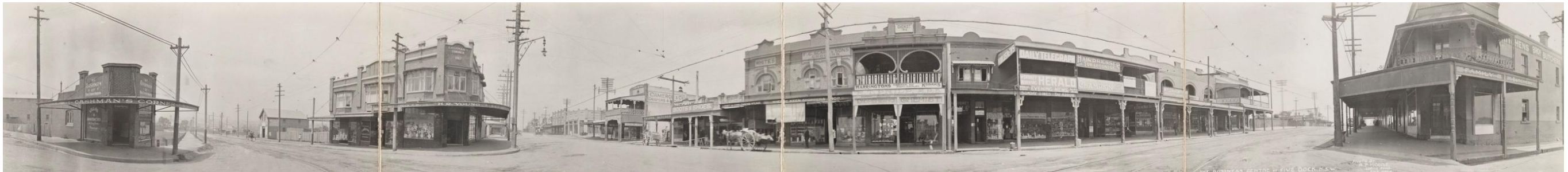
Figure 4.4 Cashman's Corner viewed from Great North Road, c1912, showing First Avenue (far left), Ramsay Road (centre) and then Great North Road (centre, right). (Source: R P Moore, SLNSW, FL8998793)
